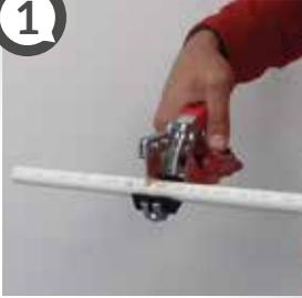
Cut the multilayer pipe right-angled with the pipe cutter.
